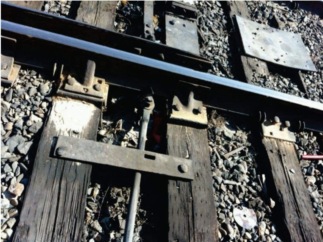
Metal Strap is an Ineffective Fix for Defect of Excessive Vertical Lateral Movement of Switch point
