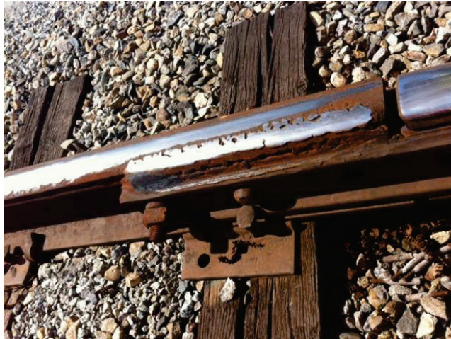
Metal Strap is an Ineffective Fix for Defect of Excessive Vertical Lateral Movement of Switch point
