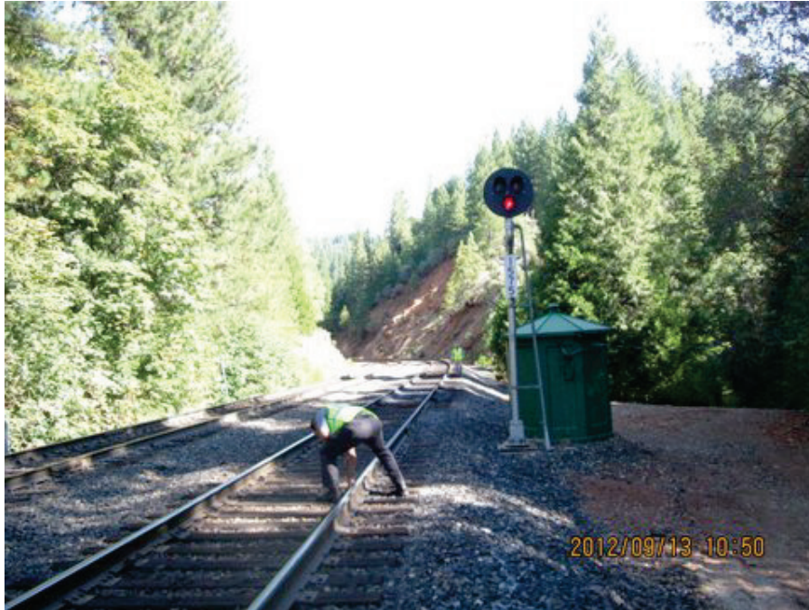
A UPRR Manager of Operating Practices (MOP) places shunts and validates the signal aspect for an FTX test in order to stop west bound Amtrak train #5 at MP 157.5 as part of a structured FTX stop test.
