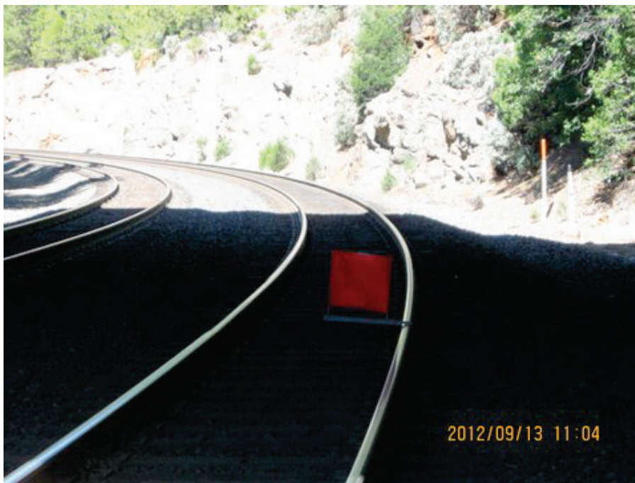
A red flag is placed about 1.2 mile downhill from a red signal at MP 157.5 on Roseville Subdivision. The flag is placed below the red signal stop so that the testing officers can observe and test for a train operating at restricted speed.
