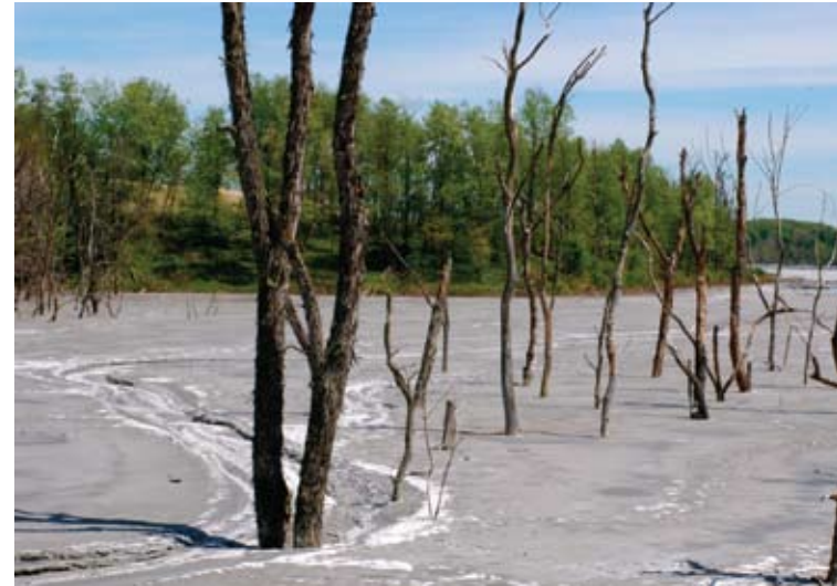
Dead trees in CCW: The Little Blue Run Residual Waste Impoundment, which straddles the border between Beaver County, PA and Hancock County, WV holds millions of tons of CCW generated by the Bruce Mansfield coal-fired power plant in Shippingport, PA. Photo credit: Mika Johnson, 2007.
