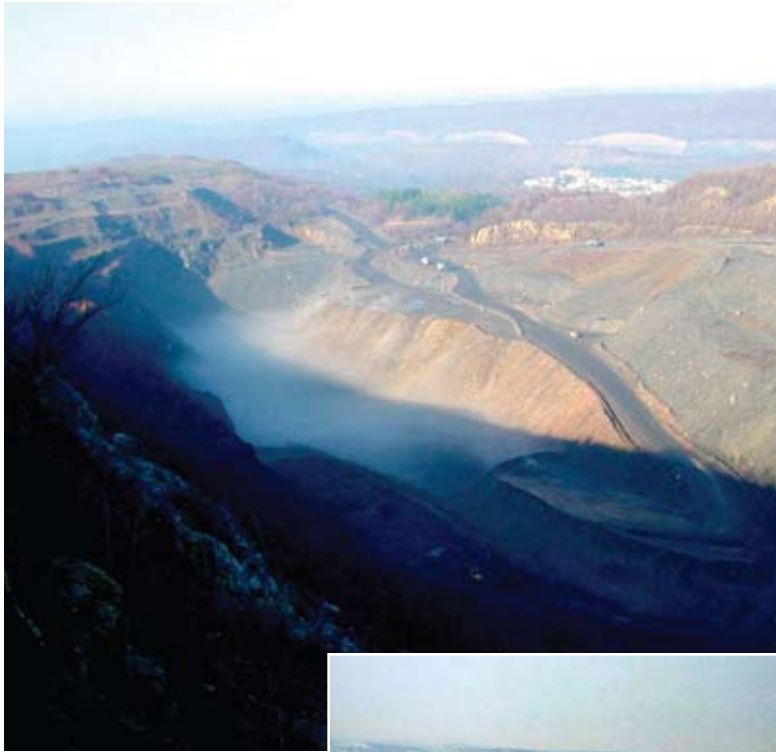
Springdale Mine Pit, Tamaqua, Pennsylvania. Photo above shows dust containing CCW rising from the mine. The immense Springdale Pit measures 700 feet deep, 1,500 feet wide and 3,000 feet long.
