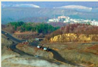
Minefill operation in Pennsylvania.
