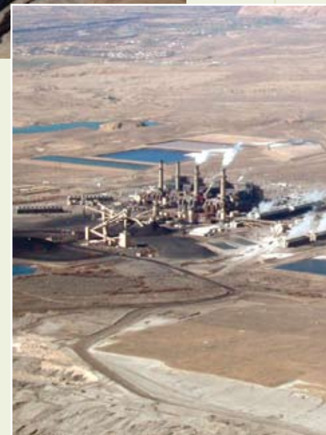
The 1,798-MW San Juan Generating Station generates about 1 million tons of CCW each year. A large quantity of the CCW is disposed in the San Juan Coal Mine.
