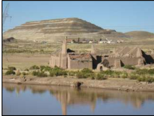
Figure 2. The large terraced hill in the background is the massive cyanide heap leach pad of Kori Kollo, which has contaminated groundwater with cyanide and other toxic pollutants over many years. Credit: Scott McKittrick (WEFTA 2011).
