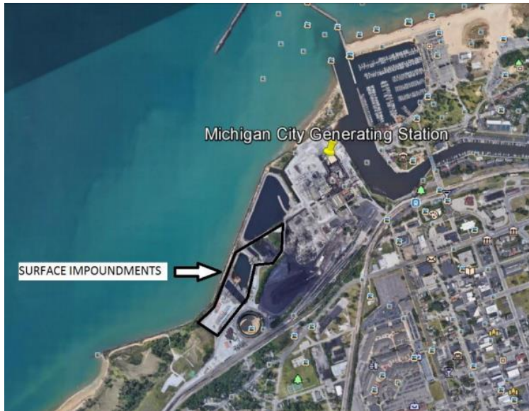
Figure 3. MCGS relative to Lake Michigan to the northwest and Trail Creek to the northeast. 23
