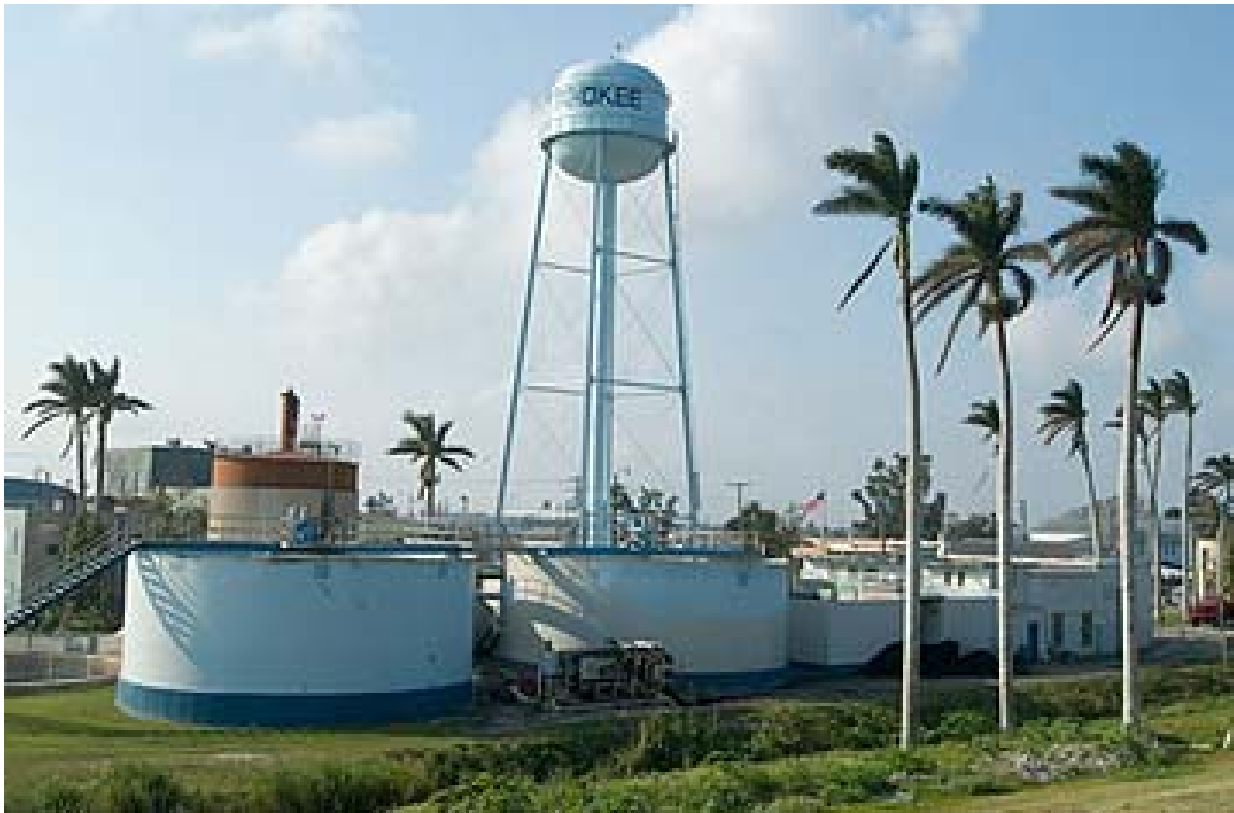
Pahokee Water Treatment Plant.
