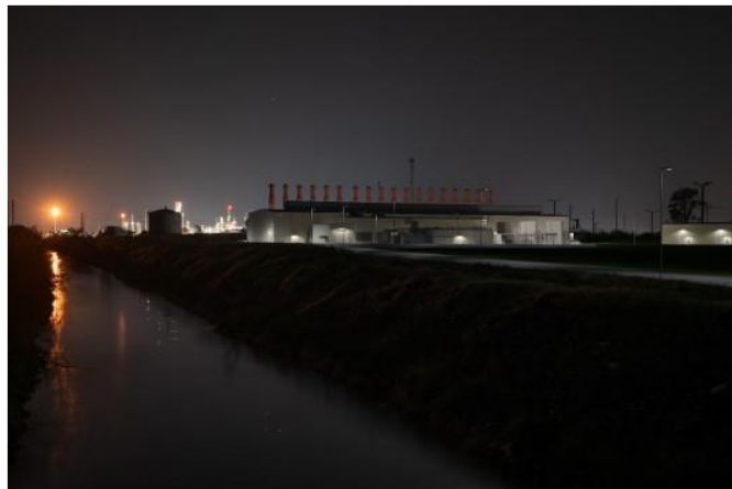
Figure 14. Entrance 02 – All lighting on.
