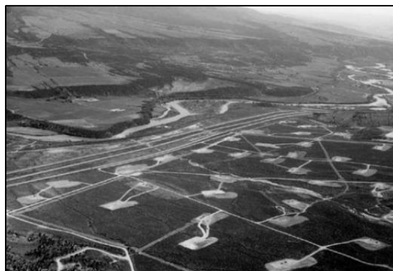
Coalbed methane infrastructure can create a dense network of well sites. Photo from Citizens Against Coalbed Methane.
