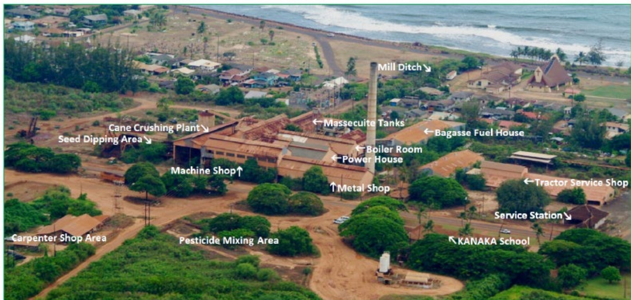
Fig. 2. Former Kekaha Sugar Mill (Source: County of Kaua‘i Office of Economic Development, FY2021 US EPA Brownfield Community-Wide Assessment Grant Application for Kekaha, Kaua‘i)
