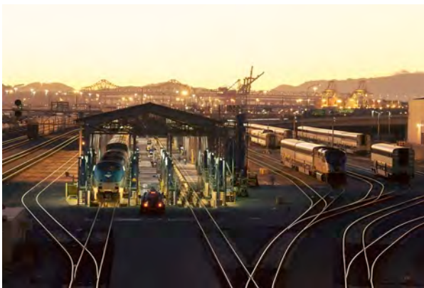
Amtrak maintenance facility in Oakland, California. With your help, Earthjustice is working with regulators and partners in California to bring the state's rail system to zero emissions. Silentfoto / Getty Images
