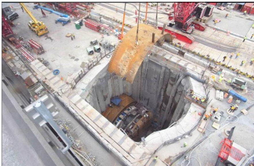
Figure 5. Removal of a damaged TBM from a temporary recovery access pit in Seattle in 2015 ( https://www.brierleyassociates.com/projects/sr99-bertha-tbm-access-shaft/ ).
