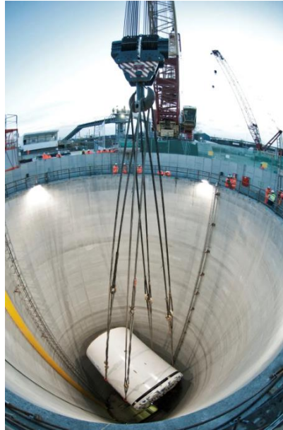
Figure 4. Use of a crane to lower a TBM section into a permanent shaft in London, England as part of a sewer interceptor boring project. Note that the L5TP shaft would be used for removing rather than deploying the Straits TBM ( https://www.ingenia.org.uk/articles/londons-deepest-tunnel-and-shafts/ ).
