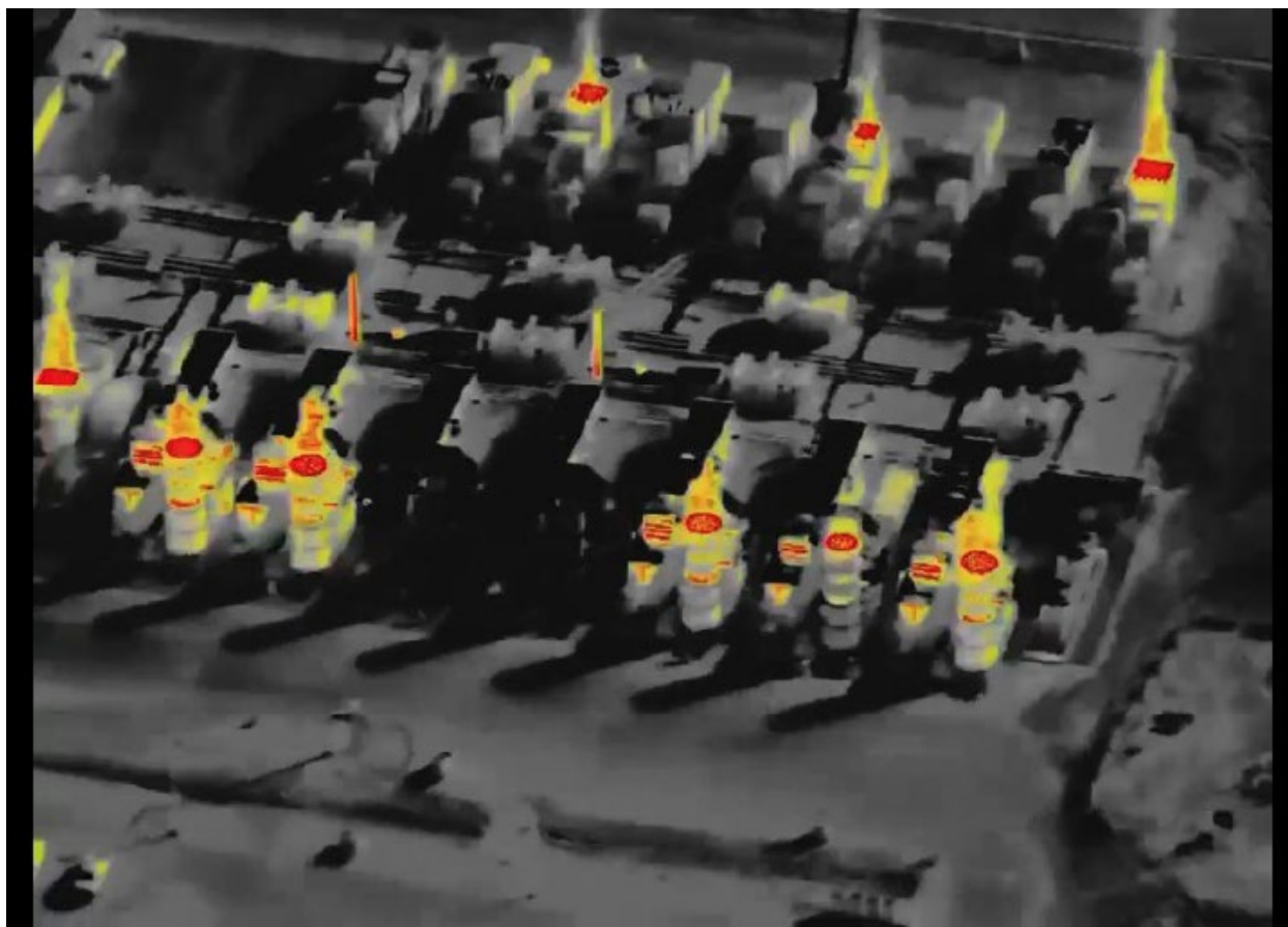
Figure 2. Thermal Camera Image of Colossus Gas Plant (Oct. 31, 2025; Steve Jones/SouthWings), Ex. D-13.
