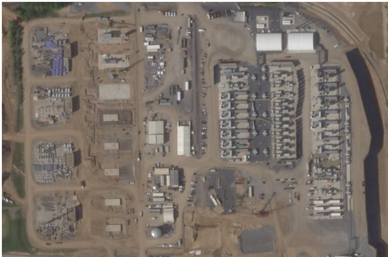
Figure 4. Close-up satellite image of Colossus Gas Plant showing twenty-seven gas-fired combustion turbines (Apr. 7, 2026), Ex. D-11.
