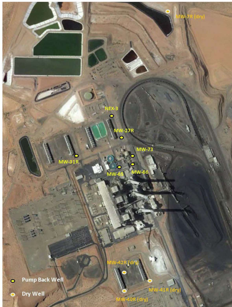
Figure 11: Carmel Formation Groundwater Recovery and Monitoring Wells (Source: Modified from Figure 1, SRP, 2016b)
