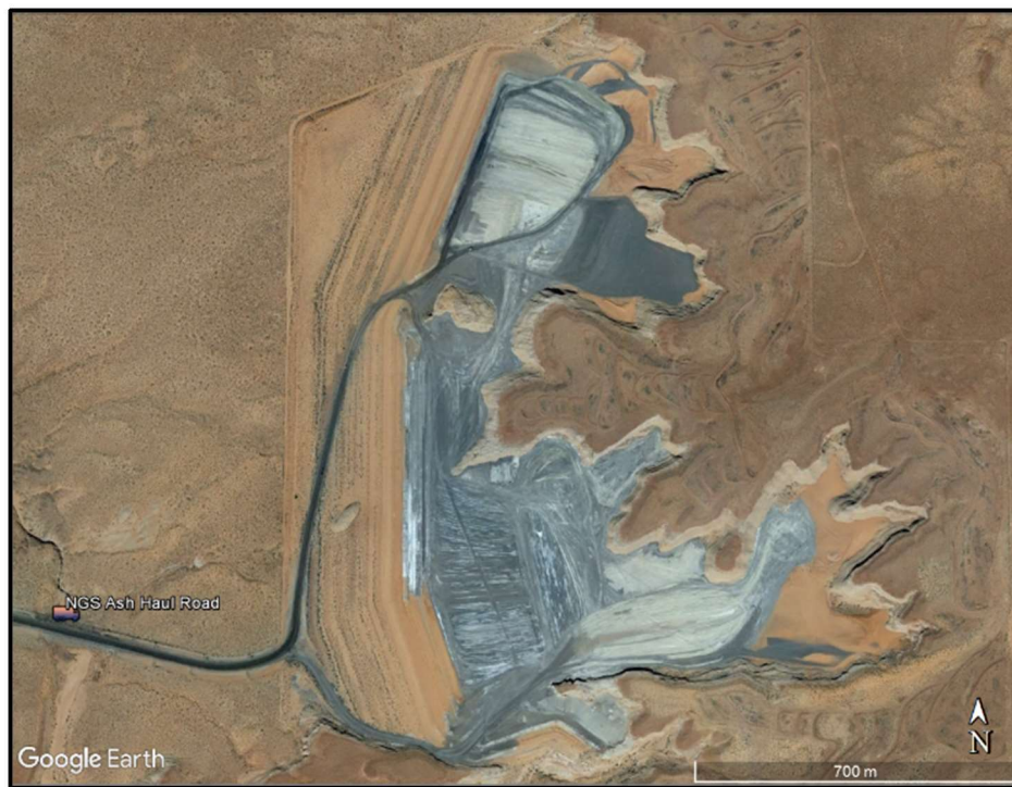
Figure 4: View of the NGS Coal-Ash Disposal Site in April of 2015 (Source: Google Earth)
