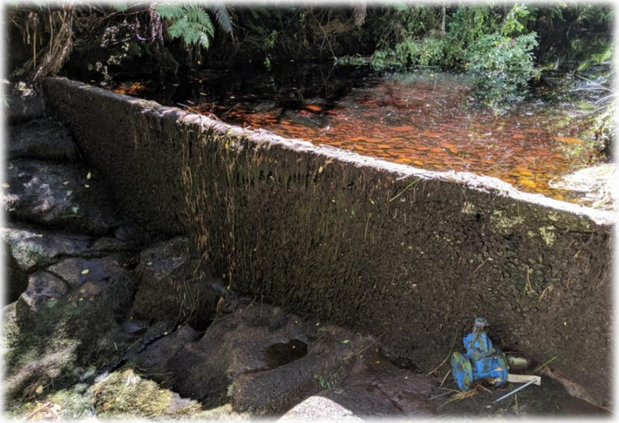
East Kawela Dam and Intake
