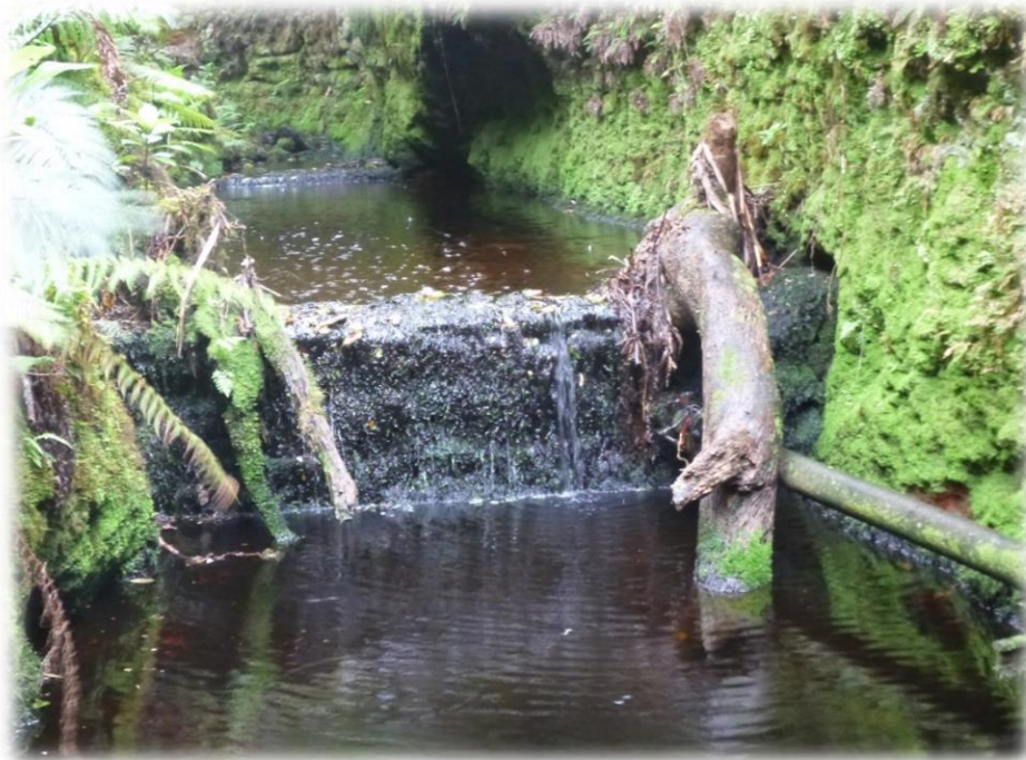
The Ranch’s Hanalilolilo diversion on Waikolu Stream
