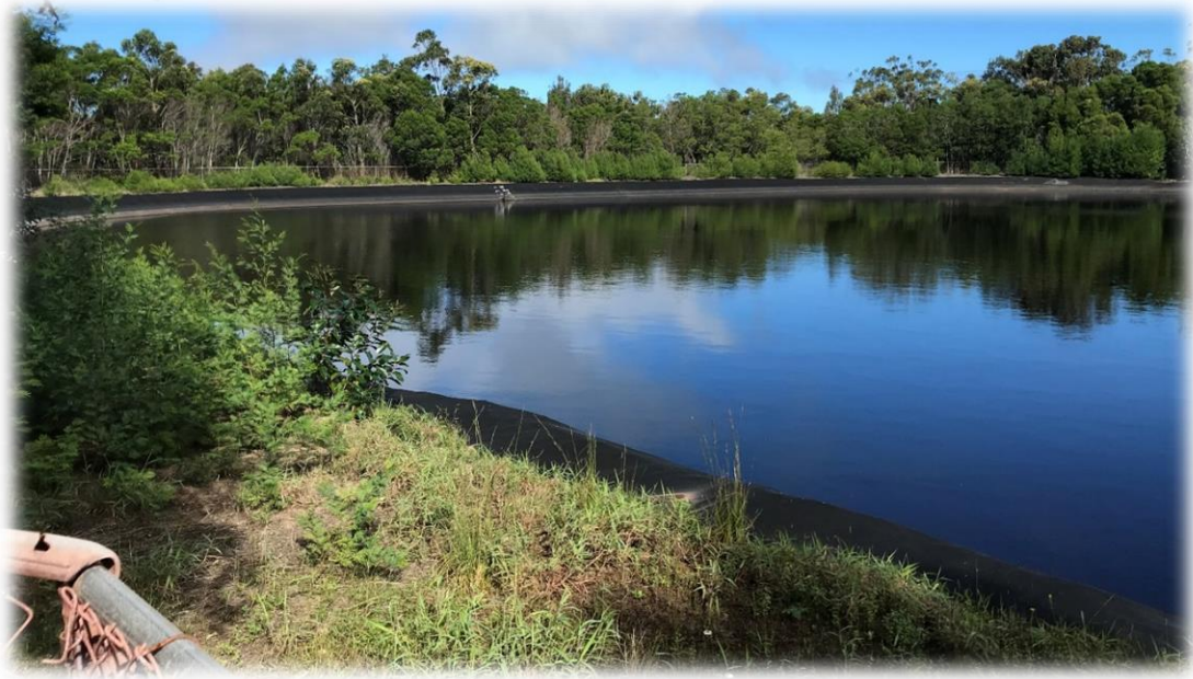
New reservoir installed in 1998, currently filled (see schematic at page 33 and Ex. 7)
