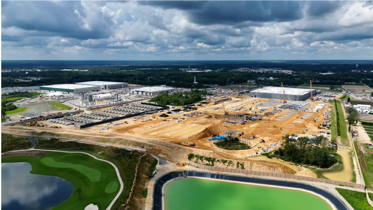
Figure 2: Aerial view of DataOne construction. (Aug. 27, 2026, Evan Simon / Floodlight)
