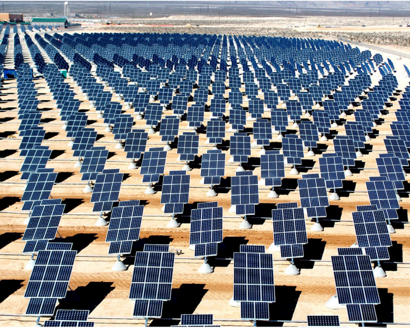
Nellis Solar Power Plant located within Nellis Air Force Base, northeast of Las Vegas, Nevada, United States. The power plant occupies 140 acres, contains about 70,000 solar panels and generates 14 megawatts of solar power for the base.
