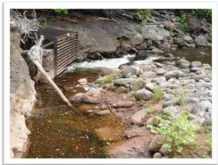
Koai'e diversion, looking from top of dam
