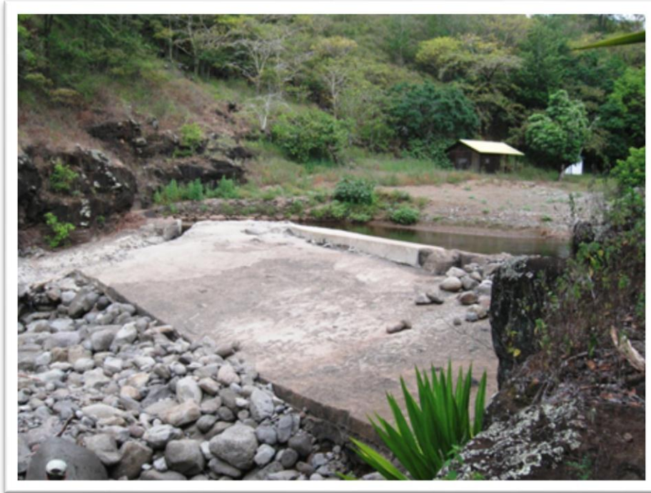
Waiahulu Dam, view from east
