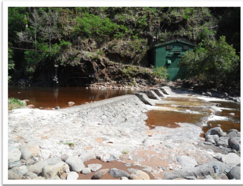
Mauka Powerhouse Dam
