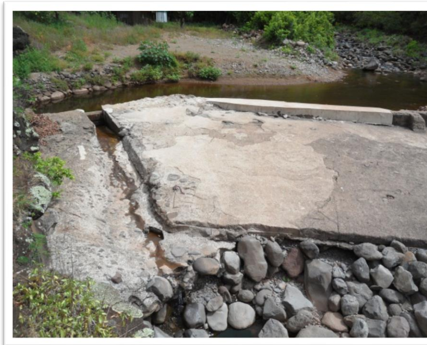
Waiahulu Dam (boarded-up outlet in middle left)
