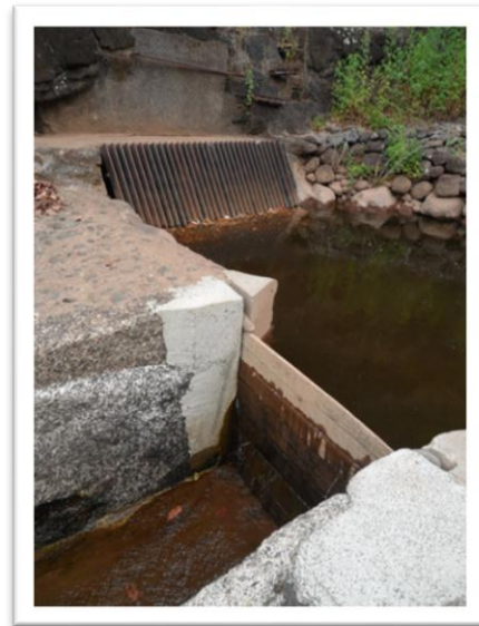
Waiahulu Dam diversion grate and boarded-up outlet
