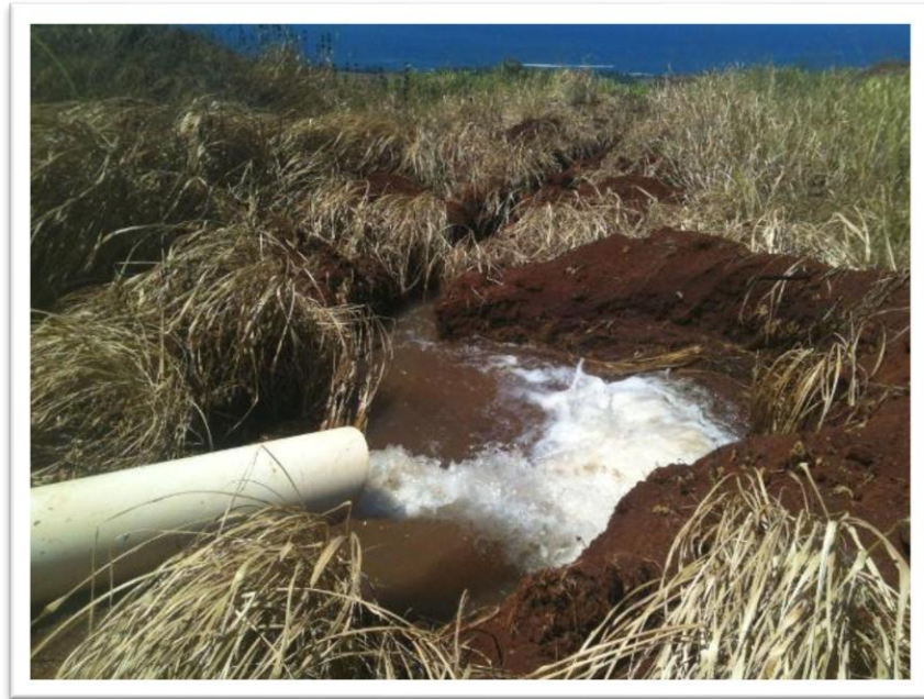
Redirected dumping from Kōke'e Ditch
