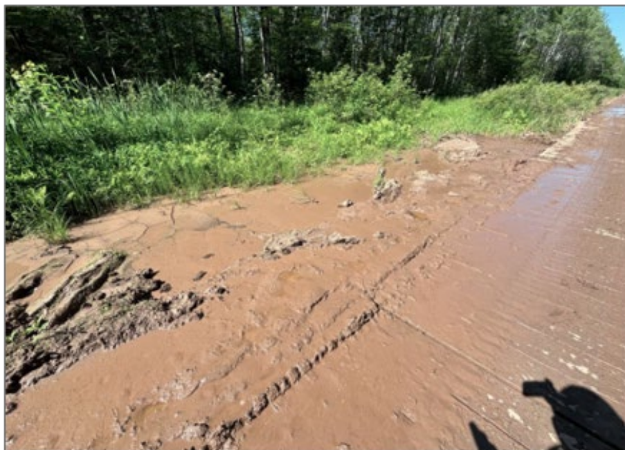
Figure 1: Soils and sediment displaced by construction matting access road being discharging into a nearby wetland at the Enbridge Check Valve Project on the Bad River Reservation (summer 2024)
