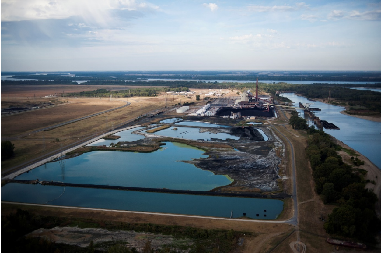
The Tennessee Valley Authority’s Allen Fossil Plant, outside of Memphis, TN, stopped burning coal in 2018. TVA is deciding whether to excavate the ash or leave it in place.
