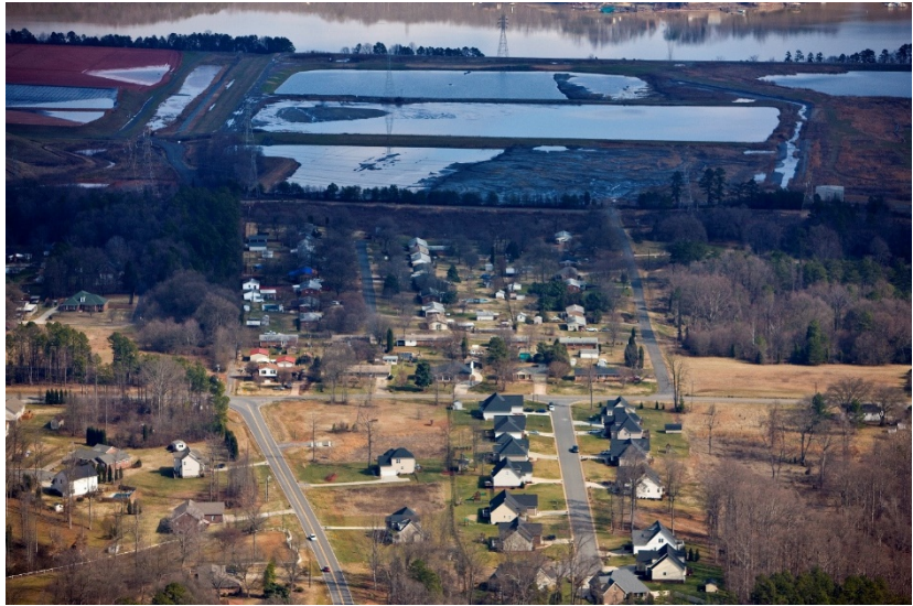
The Allen Steam Station, owned and operated by Duke Energy, is located in Belmont, NC, on the banks of the Catawba River (Lake Wylie). The coal ash dumps were built beneath the water table and are leaking toxic contaminants.
