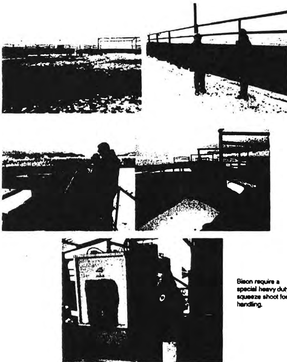
Figure 4. Bison handling facilities. The structure is 8' in height and constructed with 2 3/8" steel pipe for horizontal supports and 3" steel pipe for vertical supports.
