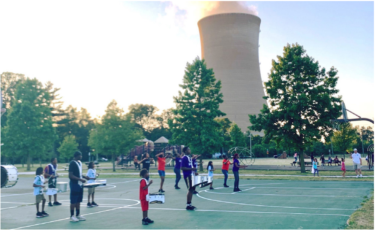
Cooling tower at the Michigan City Generating Station, Michigan City, IN. Permission from Just Transition NWI
