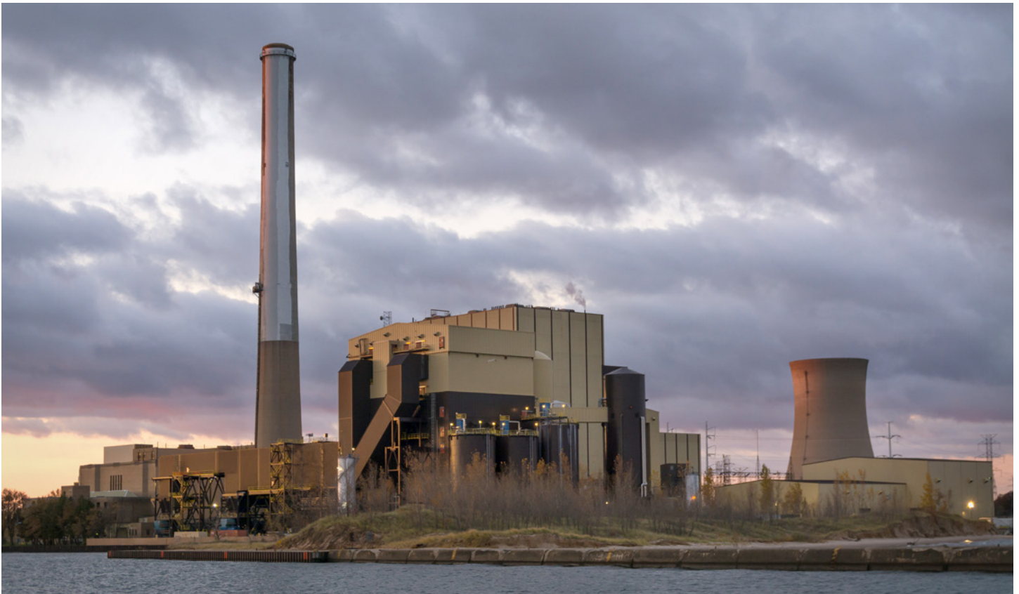
Michigan City Generating Station on Lake Michigan at sunrise, Michigan City, IN. Photo by EJ Rodriguez / Getty Images
