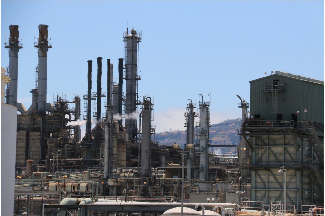
Phillips 66 refinery in California. Source: John F. Gannon.
