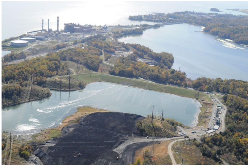
An aerial view of Dominion Virginia Power's coal ash pond at Possum Point.
