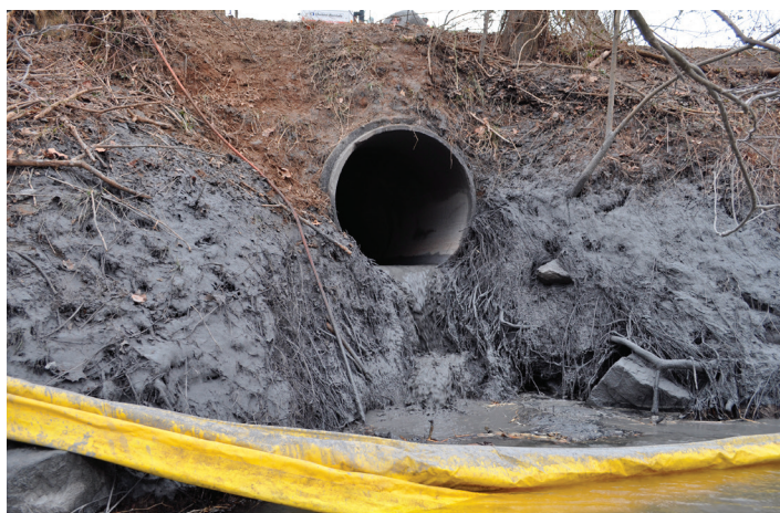
COAL ASH SPILLS FROM A STORMWATER PIPE INTO THE DAN RIVER. CREDIT: APPALACHIAN VOICES
