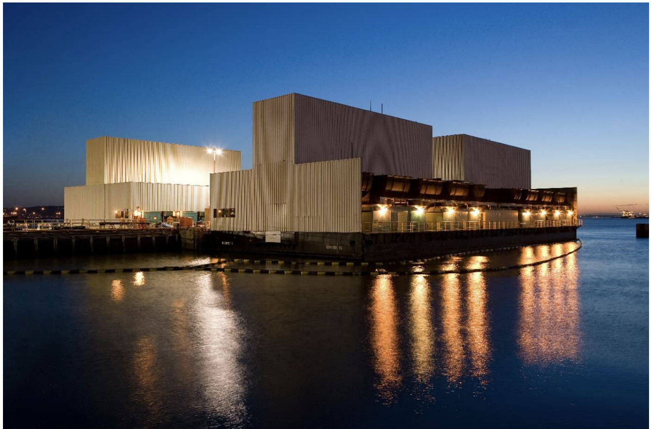
Fig. 8: Photograph of Narrows Generating Station
