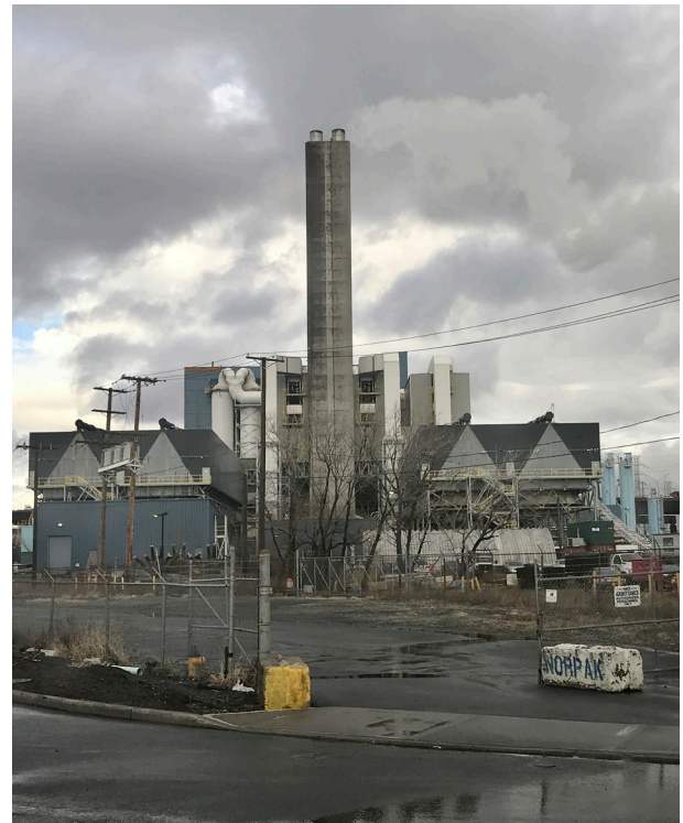
Covanta Essex incinerator in Newark, NJ. Jonathan Smith / Earthjustice
