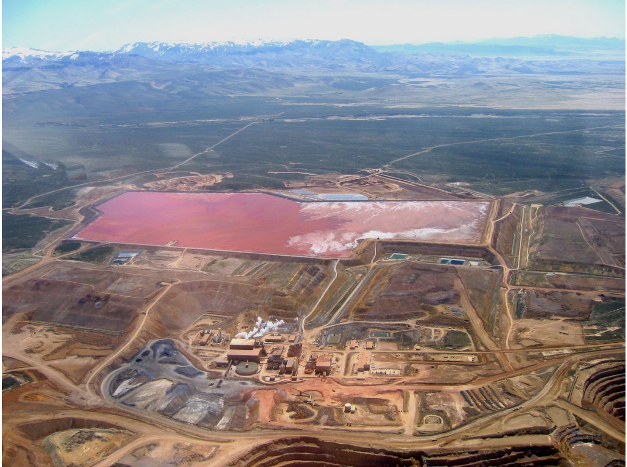
The Twin Creeks Mine, Humboldt County, Nevada. This mine uses cyanide leaching to extract gold. The red object in the photo is the surface of the tailings pond water, which is not covered. The edge of one of the mine pits appears in the bottom right side of the photo. Since this photo was taken, the tailings pond has been expanded further.
