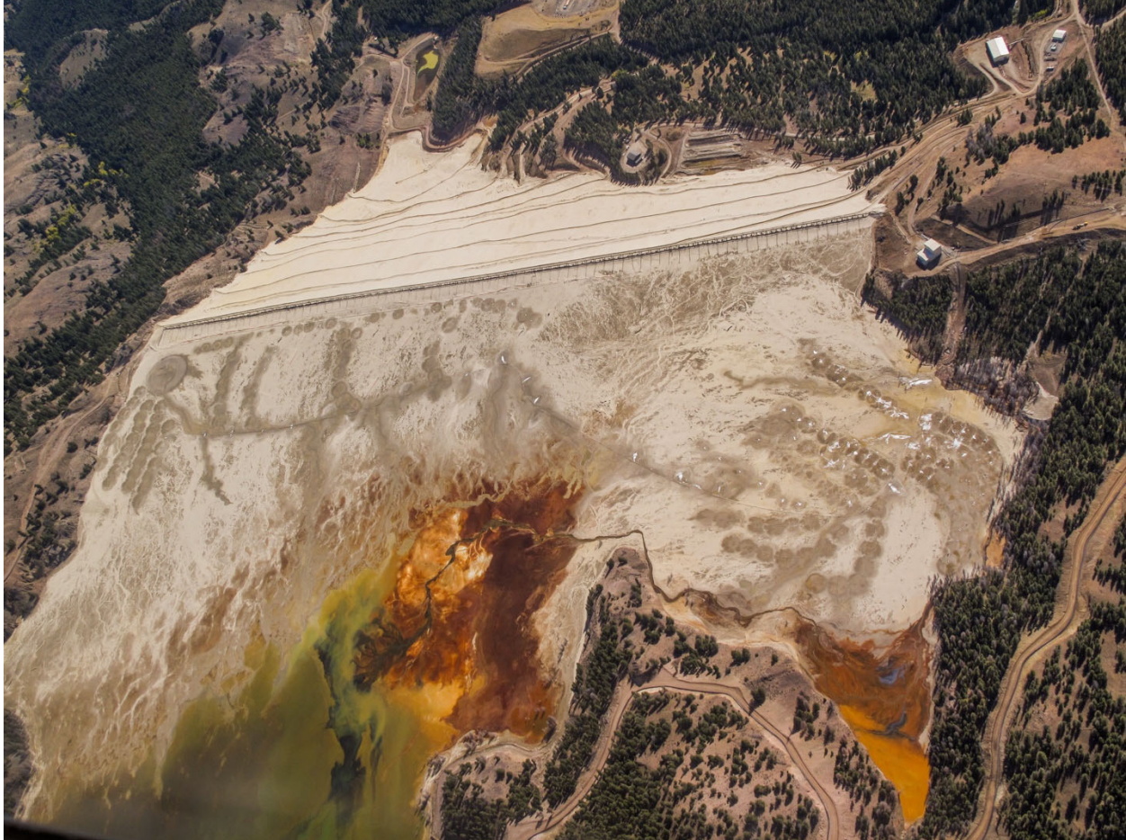
Tailings impoundment at the Thompson Creek Mine in Idaho. The lighter beige object toward the top of the photo is a 600-foot-tall sand dam holding back tailings that would otherwise spill into the Salmon River. Research shows that the number of catastrophic failures at tailings impoundments like these is increasing globally.
