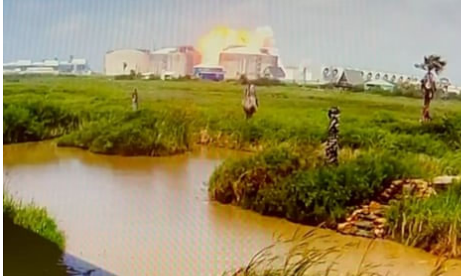
Figure 7. Photograph of explosion at Freeport LNG export terminal. 202
