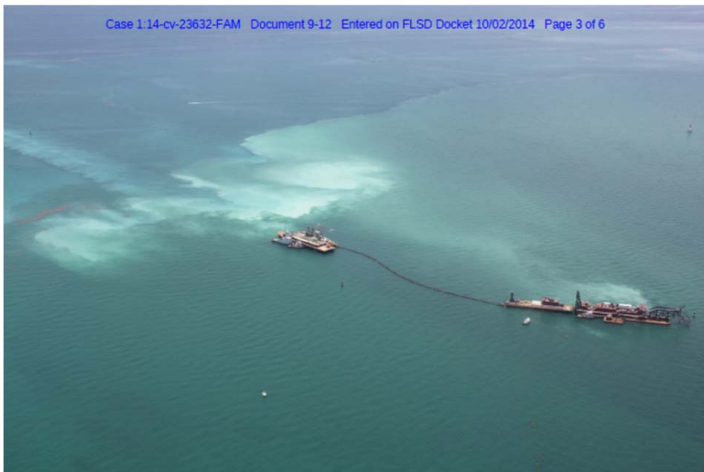
Exhibit from PortMiami litigation showing aerial view of dredging operations and sediment plumes
