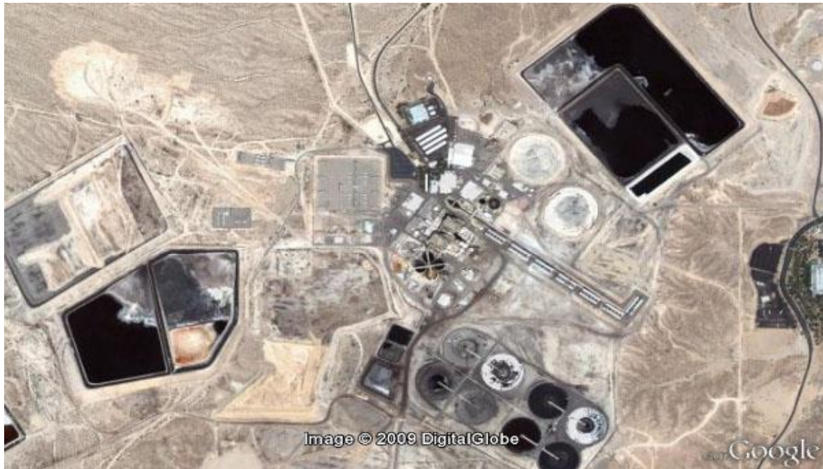
Mohave Power Plant with coal ash ponds.
